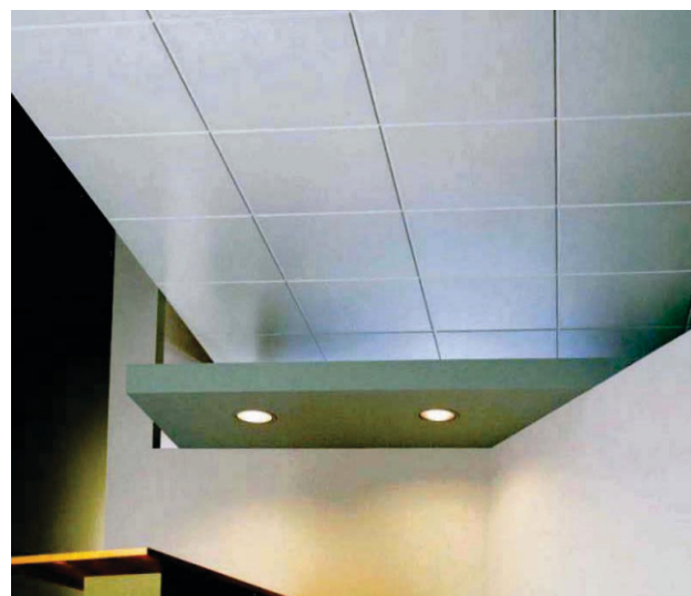
Acoustic Ceiling Installation
